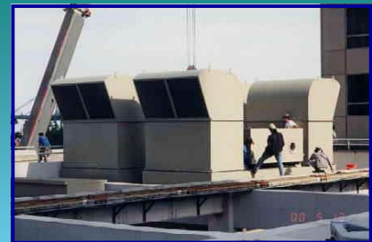
1000kVA generator sets with 70dBA @ 1m Sound Proof Enclosure
