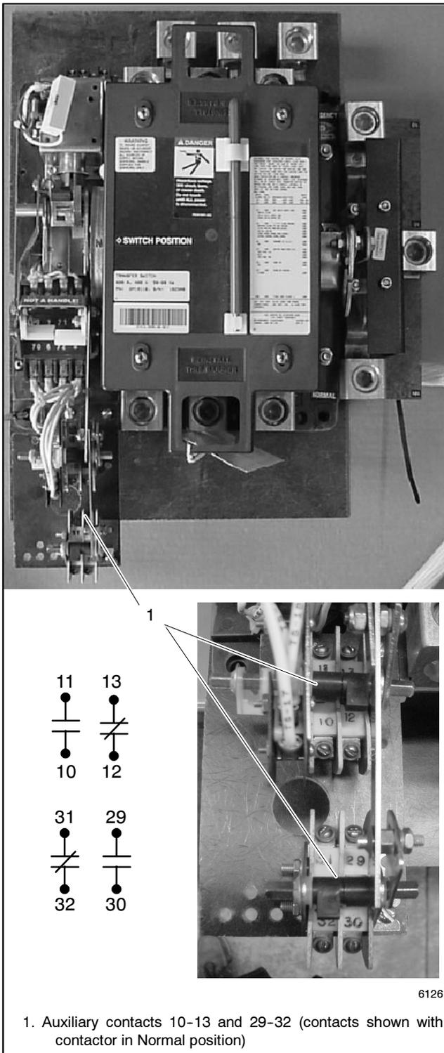
**Figure 2-26** Auxiliary Contacts, 225-400 Amp Open-Transition Models
