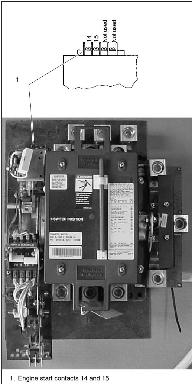
**Figure 2-22** Engine Start Contacts, 225-400 Amp Open-Transition Models
